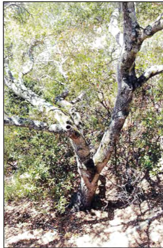
The west side of the oak, viewed from the existing deck. Some of the small cavities on branches are visible.
